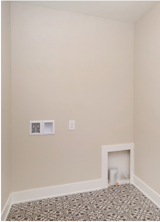
In Wall Laundry Connections
