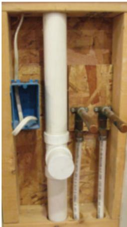
If you could peek inside your home's walls, you'd also see your plumbing pipes. For decades these were made of metal—notably copper—but today builders are finding greater reliability installing pipes made from a manmade product known as Pex™ (cross linked Polyethylene). The material has been modified for improved properties such as enhanced heat resistance and long-term strength and stability. Some
