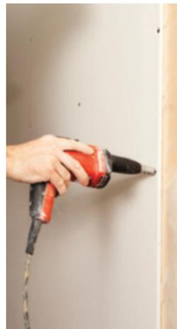
Finally, the walls themselves can offer testimony of a home's quality. Drywall panels (gypsum) can be installed using two different methods. One is to simply nail them to the framing members which, unfortunately, can cause twisting, warping and nail pops as weather begins to act on the framing members, usually made of wood. A more desirable construction method is to install drywall using glue
