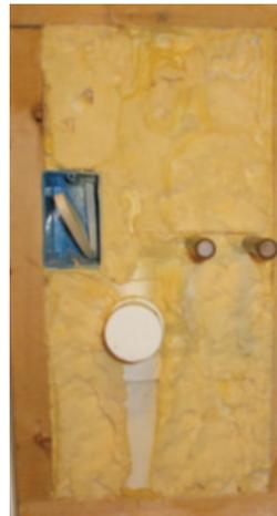
The most important thing to look for inside your walls is how well your home has been sealed. The amount and type of insulation between your walls is also important, but sealing the hundreds of small gaps and seams between framing materials, pipes, electrical boxes and other mechanical elements will help prevent unintended thermal loss. One of the most effective methods for insulation today is Icynene® foam
