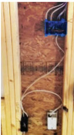
The walls of your home also conceal the electrical wiring that brings power from outside your home to the appliances and other devices inside. All wiring work is performed to strict rules and local codes which determine the types of wiring used and where it's to be placed inside your walls. After installation, but before closing the walls, the electrical system is then checked thoroughly by licensed inspectors to make
