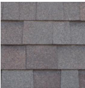
The most common type of roofing material is a composite of asphalt and fiberglass. Composite shingles come in more shapes and sizes than any other shingle, providing significant design flexibility along with durability. Over
