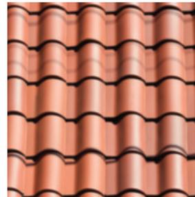
Made from clay/ceramic material, tile roofing can be extremely resilient to harsh climates, especially those with an abundance of heat and sunshine. Typically, tile roofs can reflect more than 50% of the sun's energy, working as a natural inhibitor of thermal
